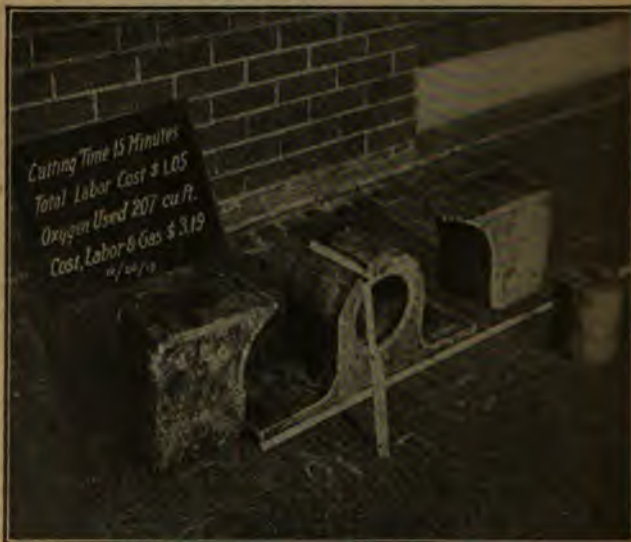
Fig. 5. A Davit Collar made with an oxy-acetylene torch.
